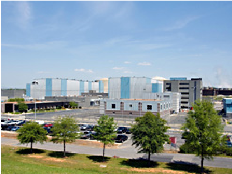
Figure 3-49: Catawba Nuclear Station
