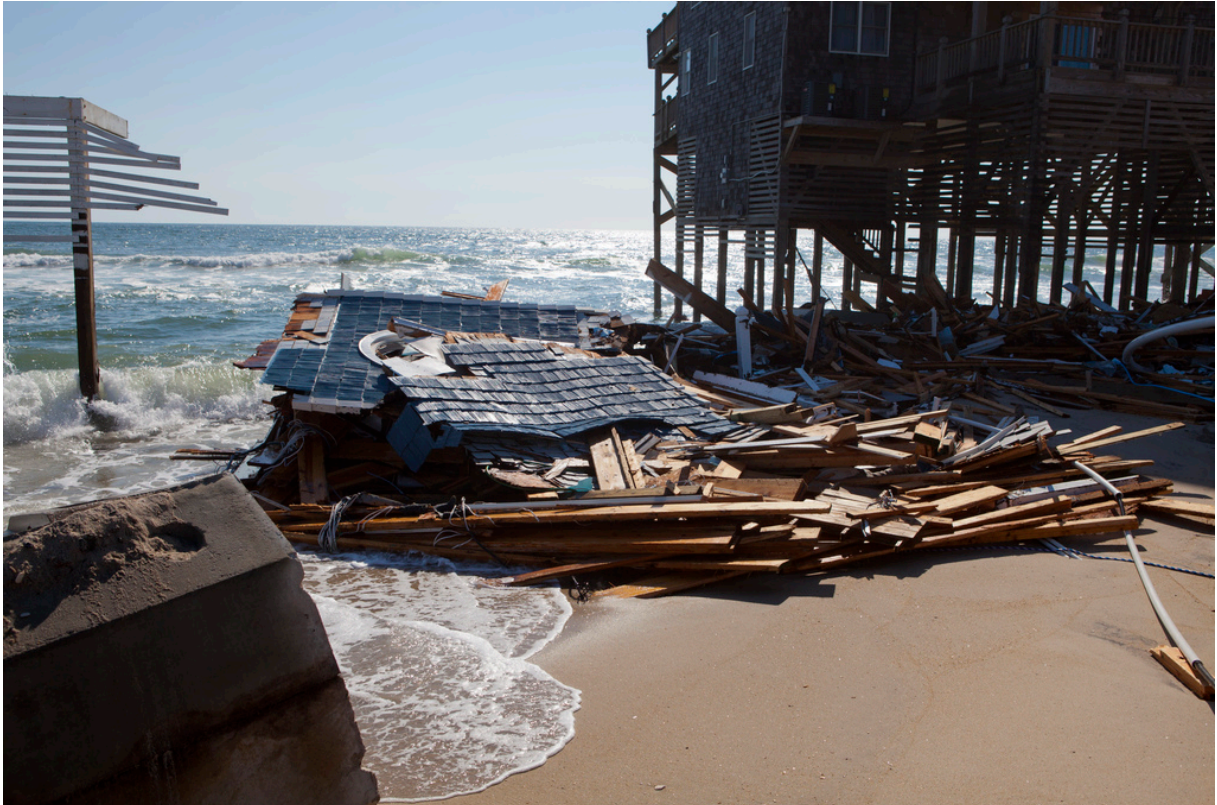
Figure 3-39 Severe Beach Erosion on North Carolina Outer Banks
