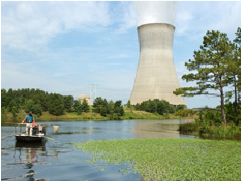
Figure 3-46: Harris Nuclear Plant
